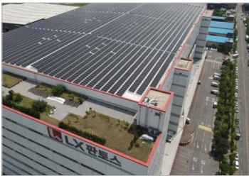
View of the solar power generation facility installation
