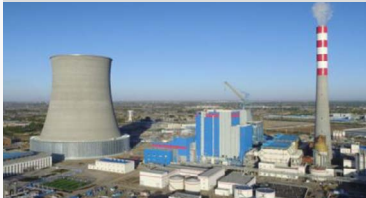
Wuwei cogeneration plant
