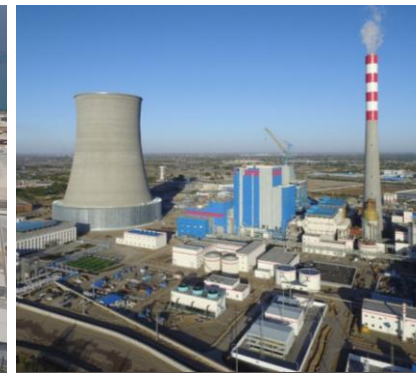
Wuwei CHP Plant
