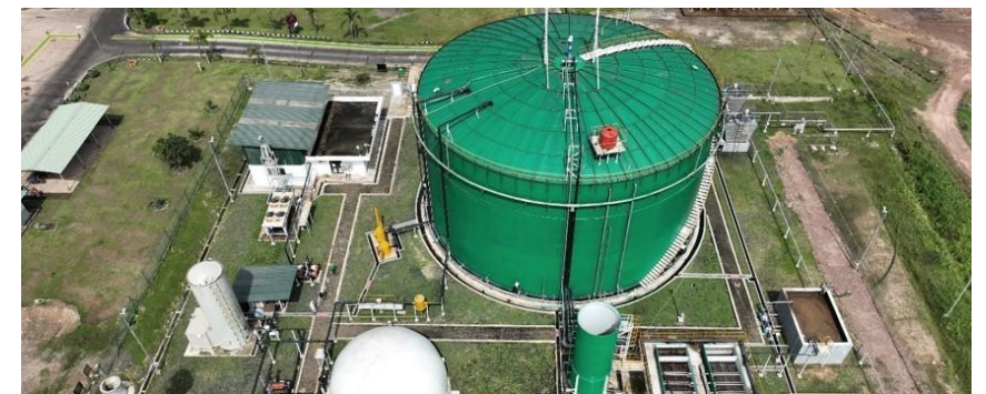
Biogas Power Plant at TBSM, Indonesia
