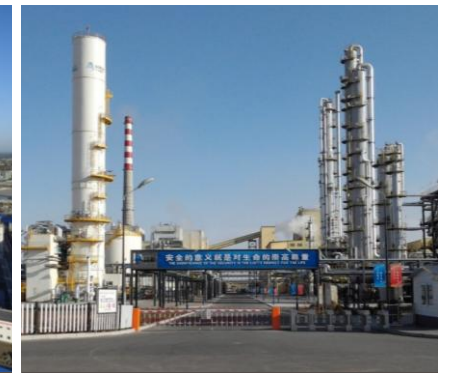
Inner Mongolia Urea Plant
