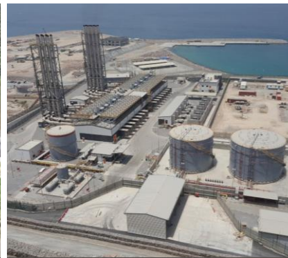
Musandam Gas Power Plant
