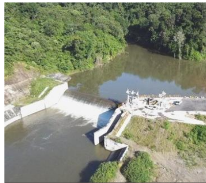
Hasang Hydropower Plant
