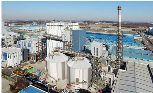
Poseung Biomass Power Plant
