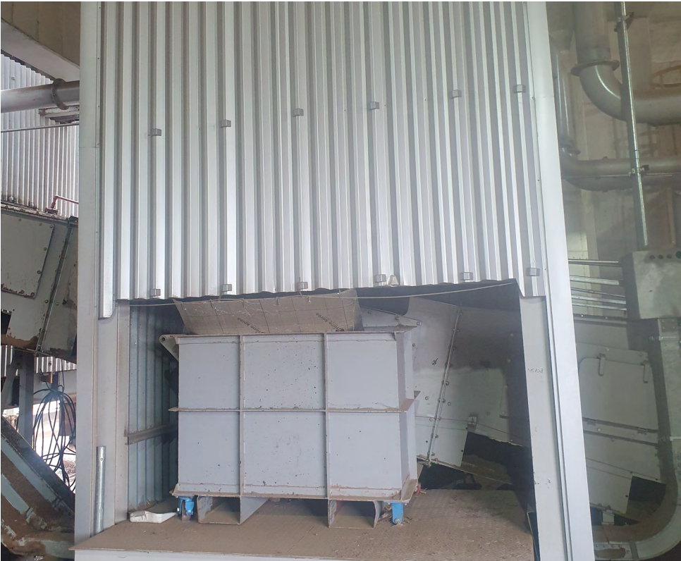
Magnetic Separator: A device that separates magnetic materials from a mixture by attracting only substances that respond to a magnetic field.
